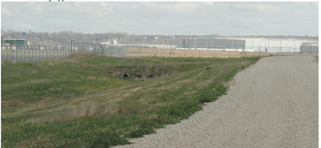
Fig 3. View of Culvert No. 2., looking north. Tallgrass Archaeology LLC photograph, April 11, 2024.
