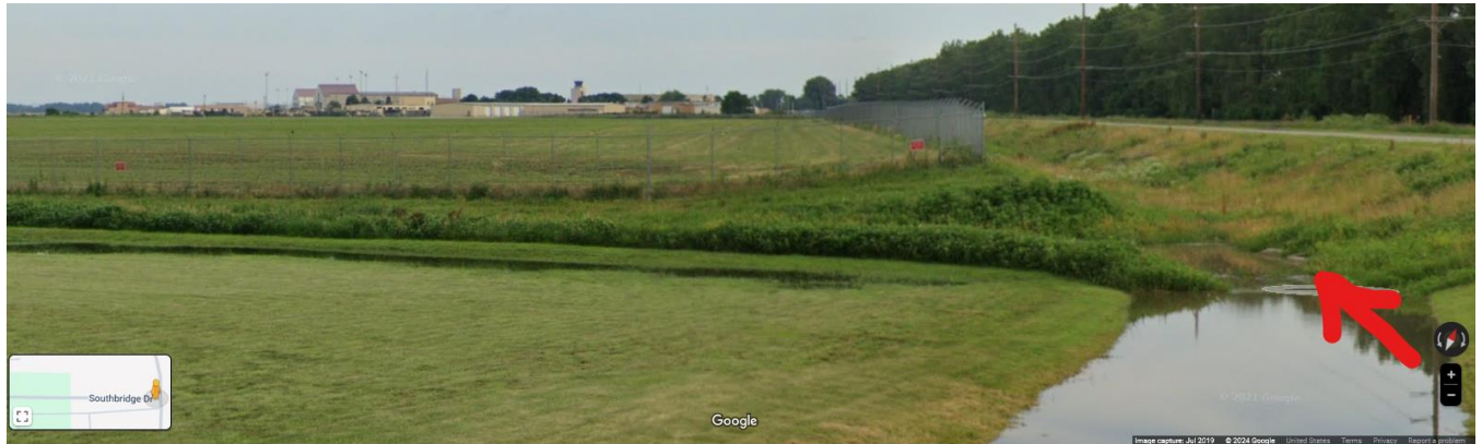
Fig 7. View of multi-culvert (No. 17) near west side of Southbridge Ave, near Sully Ave, looking north. Source: Google Street View, July 2019.
