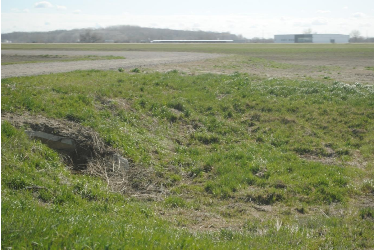
Fig 4. View of Culvert No. 4, looking east. Tallgrass Archaeology LLC photograph, April 11, 2024.
