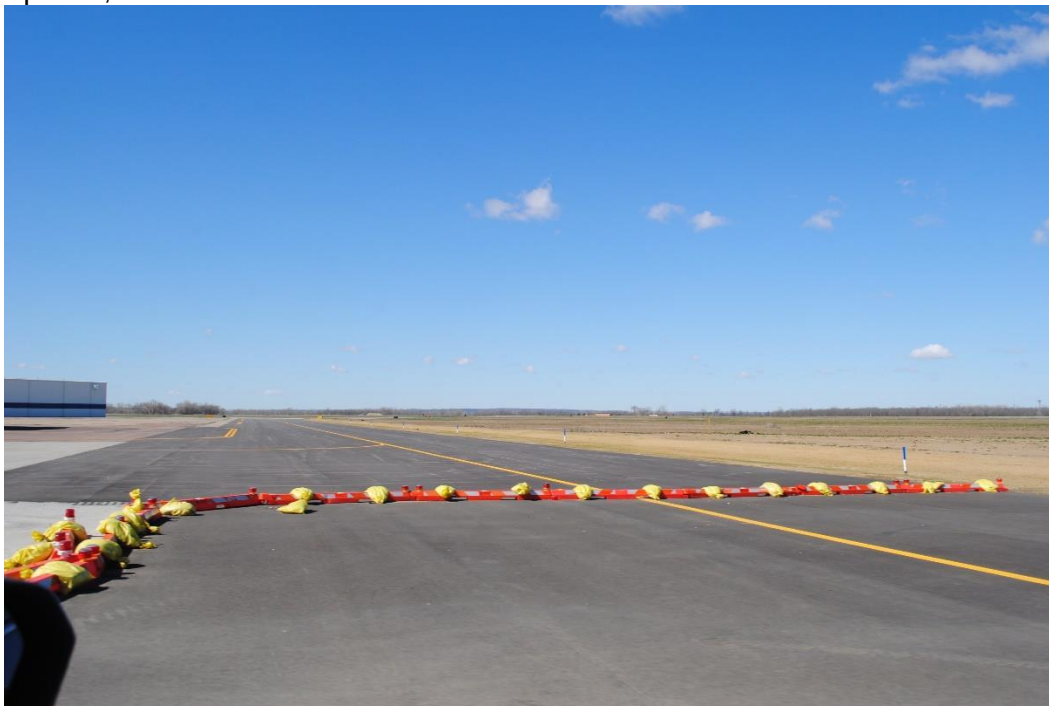
Fig 13. View of paved areas near north end of airfield. Tallgrass Archaeology LLC photograph, April 11, 2024.
