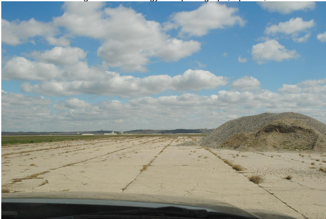
Fig 7. View of some 1950s or 1960s pavement, part of former runway that has been largely removed, looking northeast. Tallgrass Archaeology LLC photograph, April 11, 2024.
