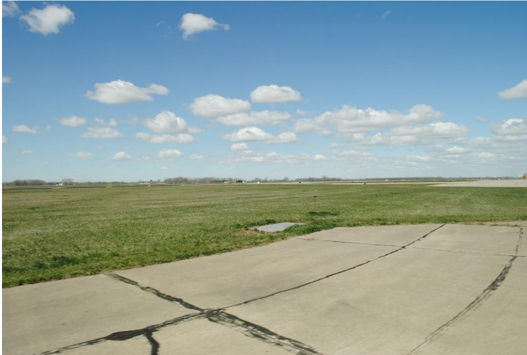
Fig 12. View of airbase apron in distance, looking northwest. Tallgrass Archaeology LLC photograph, April 11, 2024.
