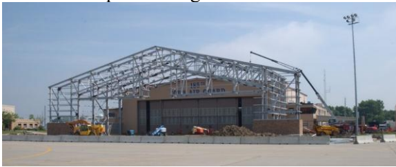
2004 photograph showing construction of the hangar's large, apron-facing side, looking north. Source: De Groot 2023.
