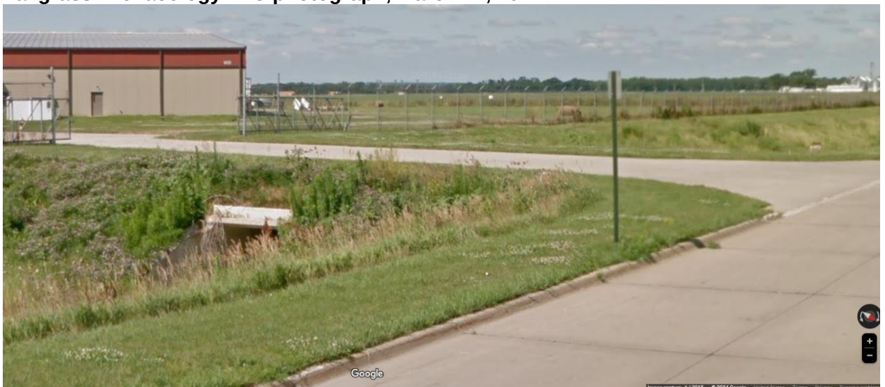
Fig 8. View of modern concrete box culvert near aviation museum, looking southwest. Source: Google Street View, July 2015.
