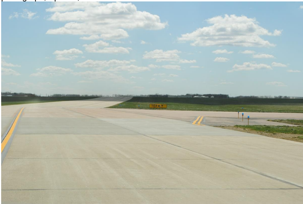
Fig 15. View of the pavement in the airfield, looking southeast. Tallgrass Archaeology LLC photograph, April 11, 2024.
