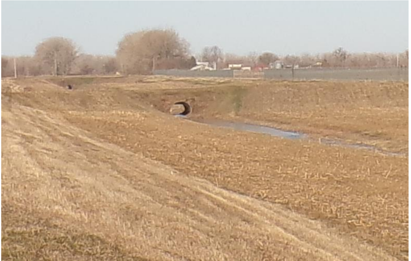
Fig 4. View of culverts No. 9 (background) and 10 (foreground), looking west. Tallgrass Archaeology LLC photograph, April 11, 2024.
