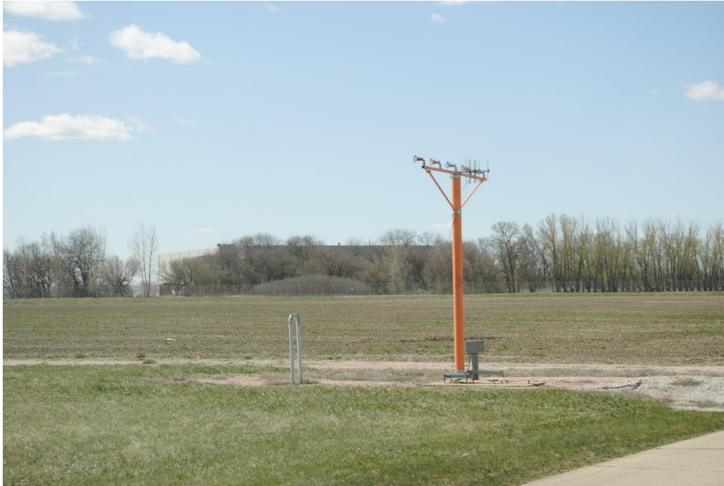
Fig 10. View of directional infrastructure, looking south from near south end of Runway 13-31. Tallgrass Archaeology LLC photograph, April 11, 2024.
