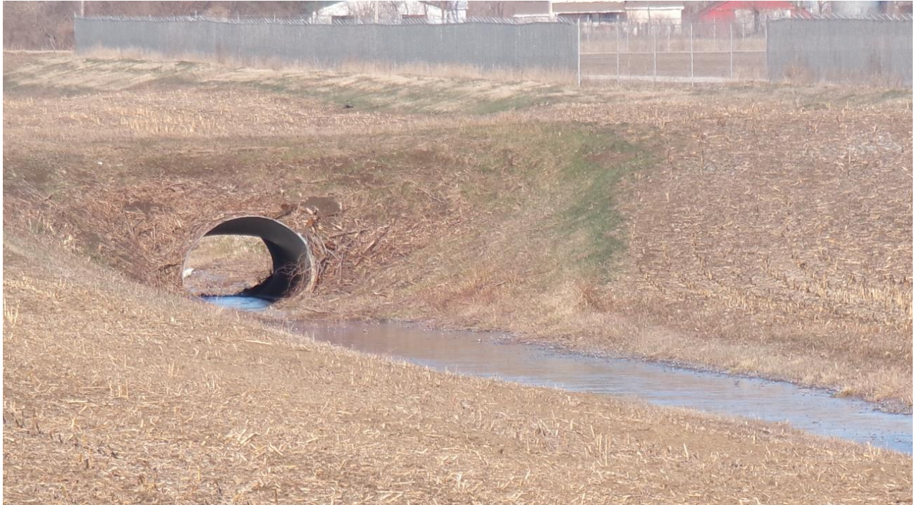
Fig 3. View of Culvert No. 10, looking west. Tallgrass Archaeology LLC photograph, April 11, 2024.
