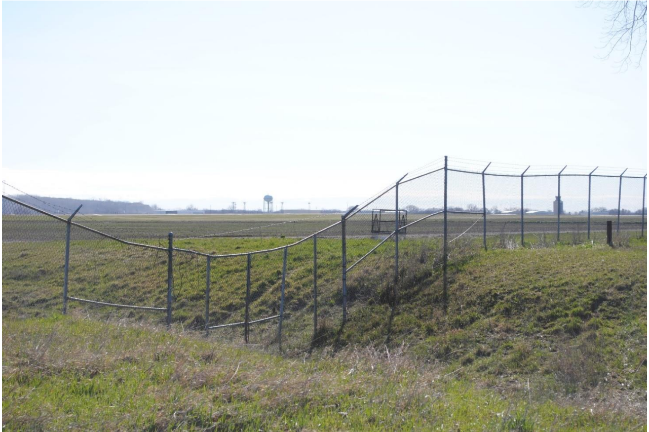
Fig 5. View of perimeter fencing across the ditch at north end of airport, looking southeast.
