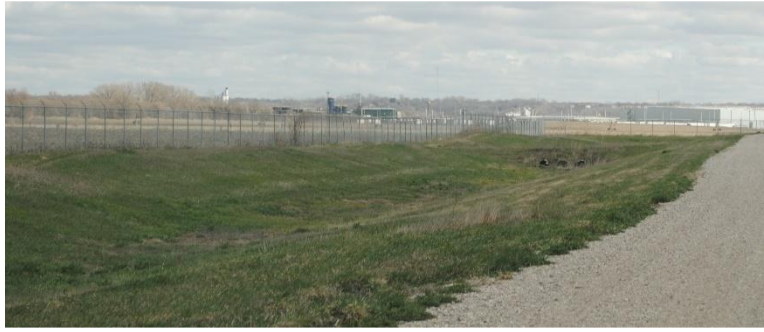
Multi-culvert and ditch west of Seaboard Triumph Pkwy, looking east.
