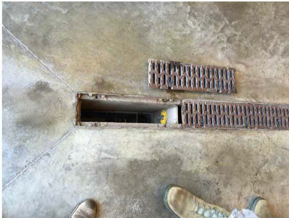
Photo 17: Trench train with drain plug in Building 286 – Current Fire Station
