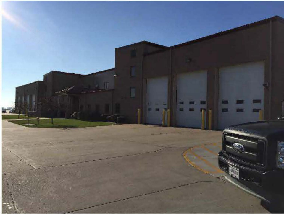
Photo 13: Building 286 – Current Fire Station
