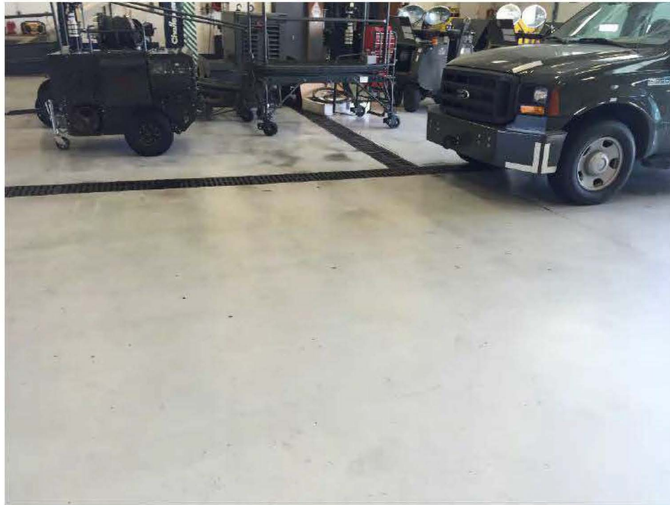
Photo 1: Trench drain in Building 252
