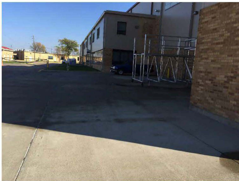
Photo 6: Northwest portion of the location where AFFF would have been pushed out of Building 261 – Main Hangar
