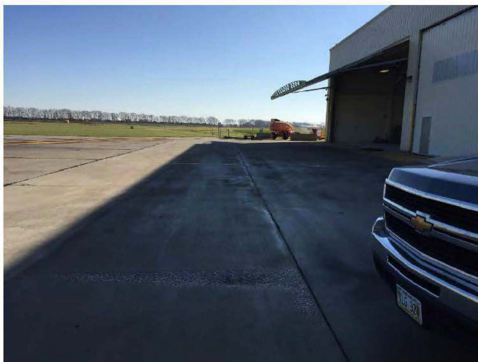
Photo 12: Concrete apron north of Building 241 – ANG Paint Facility (Bays 1 and 2)
