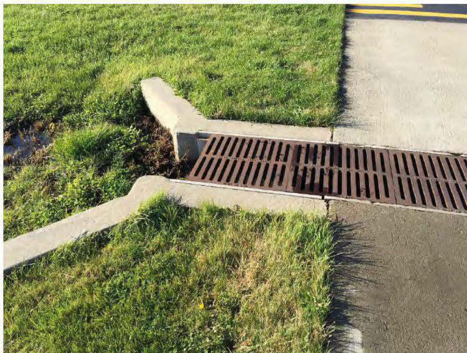
Photo 18: Trench train across drive at Building 286 – Current Fire Station (adjacent to nozzle testing area)
