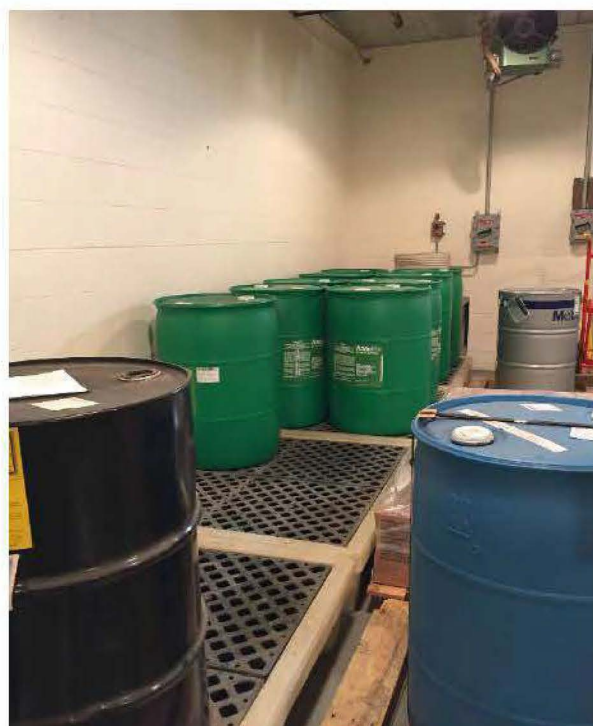
Photo 24: AFFF drum storage in Building 281 – Hazmat Pharmacy
