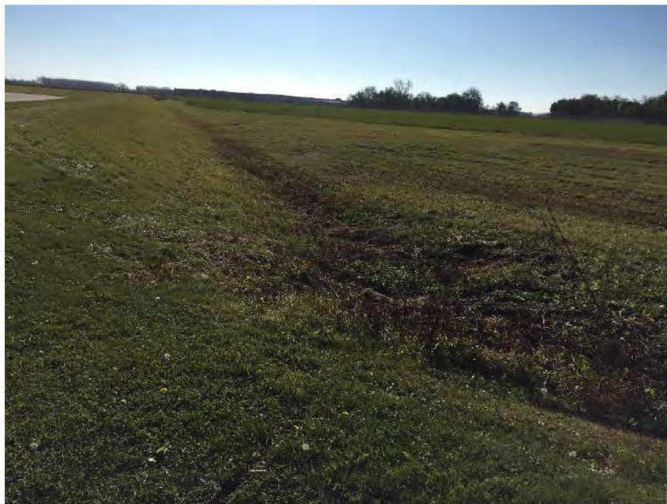
Photo 11: Ditch southeast of Building 241 – ANG Paint Facility drainage
