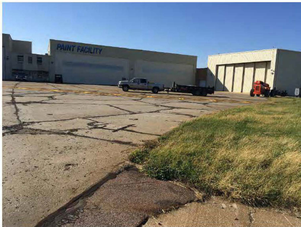
Photo 7: Building 241 – ANG Paint Facility
