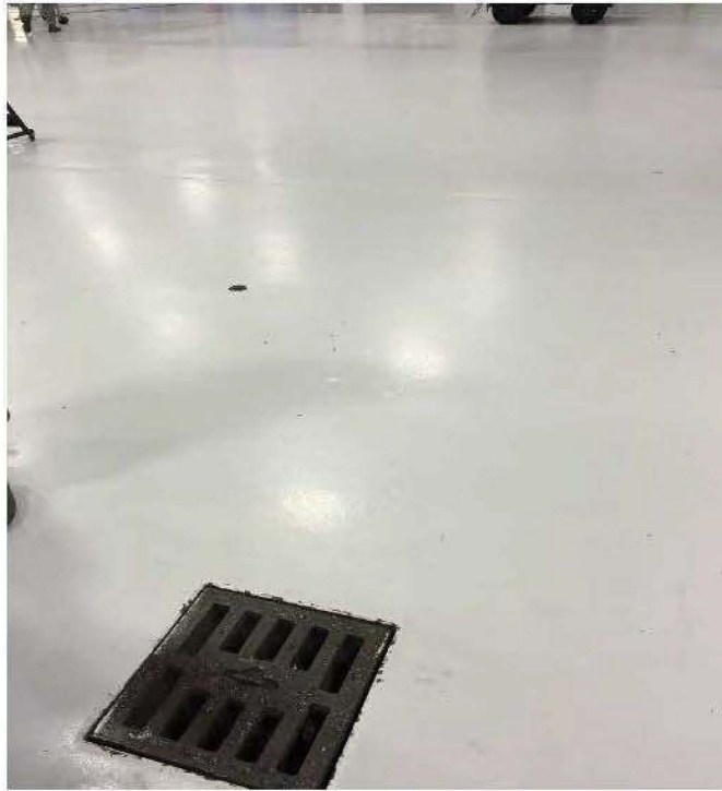
Photo 3: Floor drain in Building 261 – Main Hangar
