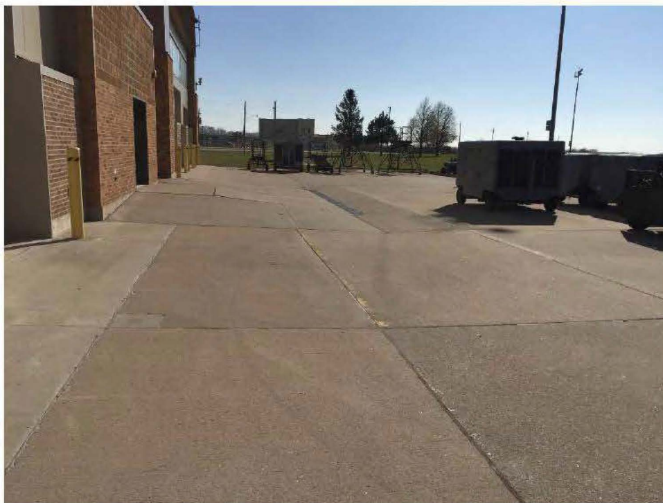
Photo 2: Location where AFFF would have been pushed out of Building 252
