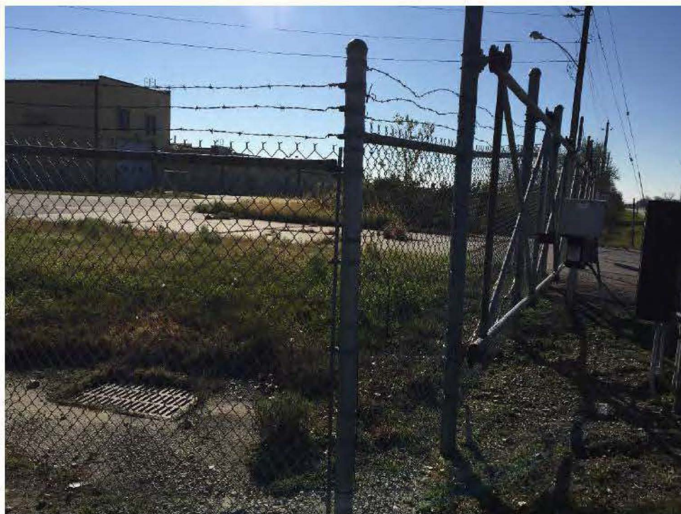
Photo 22: Stormwater Sewer System outfall (looking south where sewer daylights)
