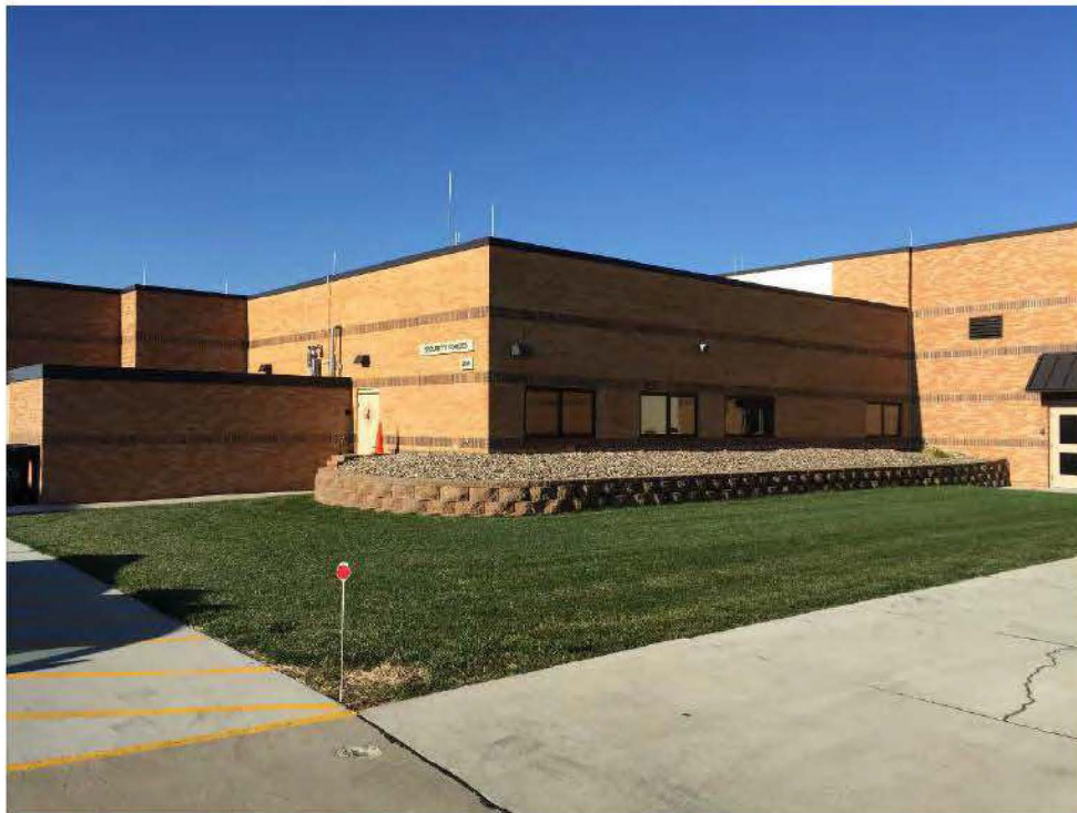
Photo 19: Building 284 – Former Fire Station (Current Security Forces Building)
